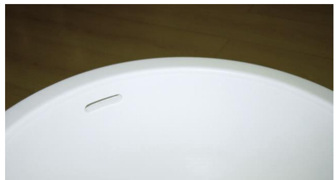
Undermounted bowl with overflow
